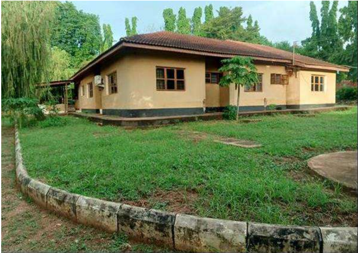
Plate 2.2: The Main building (OUT Regional Centre Office)
