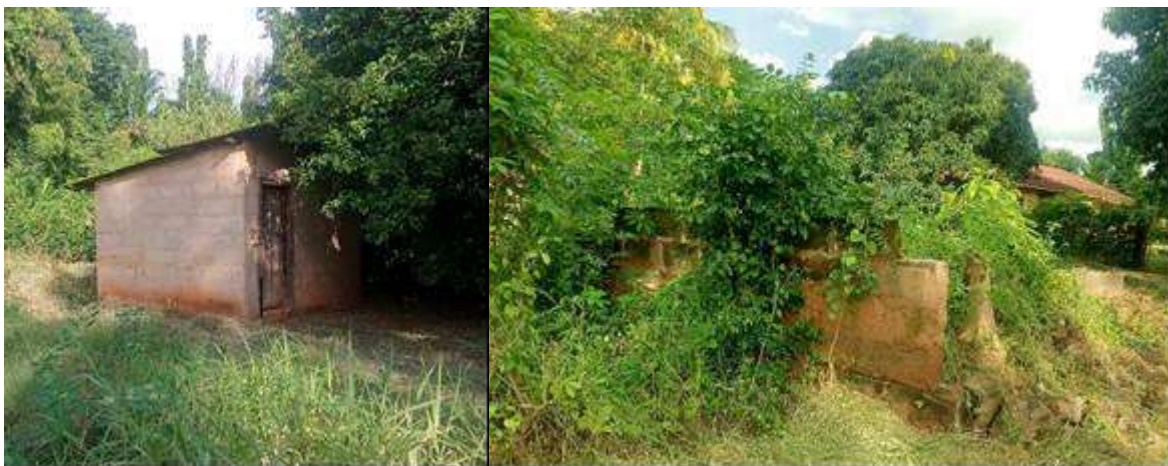
Plate 2.3: Existing structures in site
