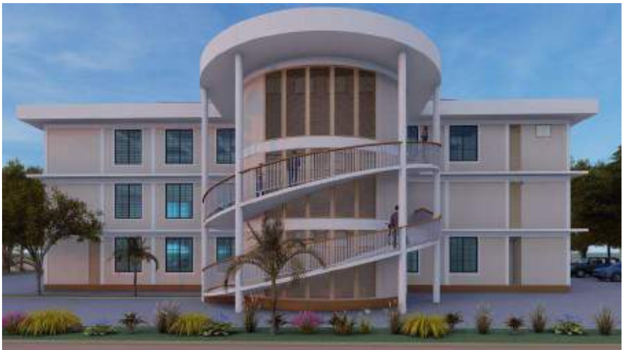
Figure 2.3: Rear view of the building
